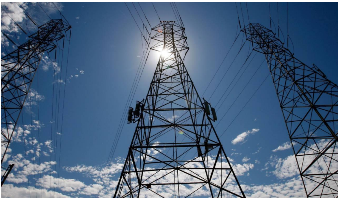
Torre electrica / Getty Images
